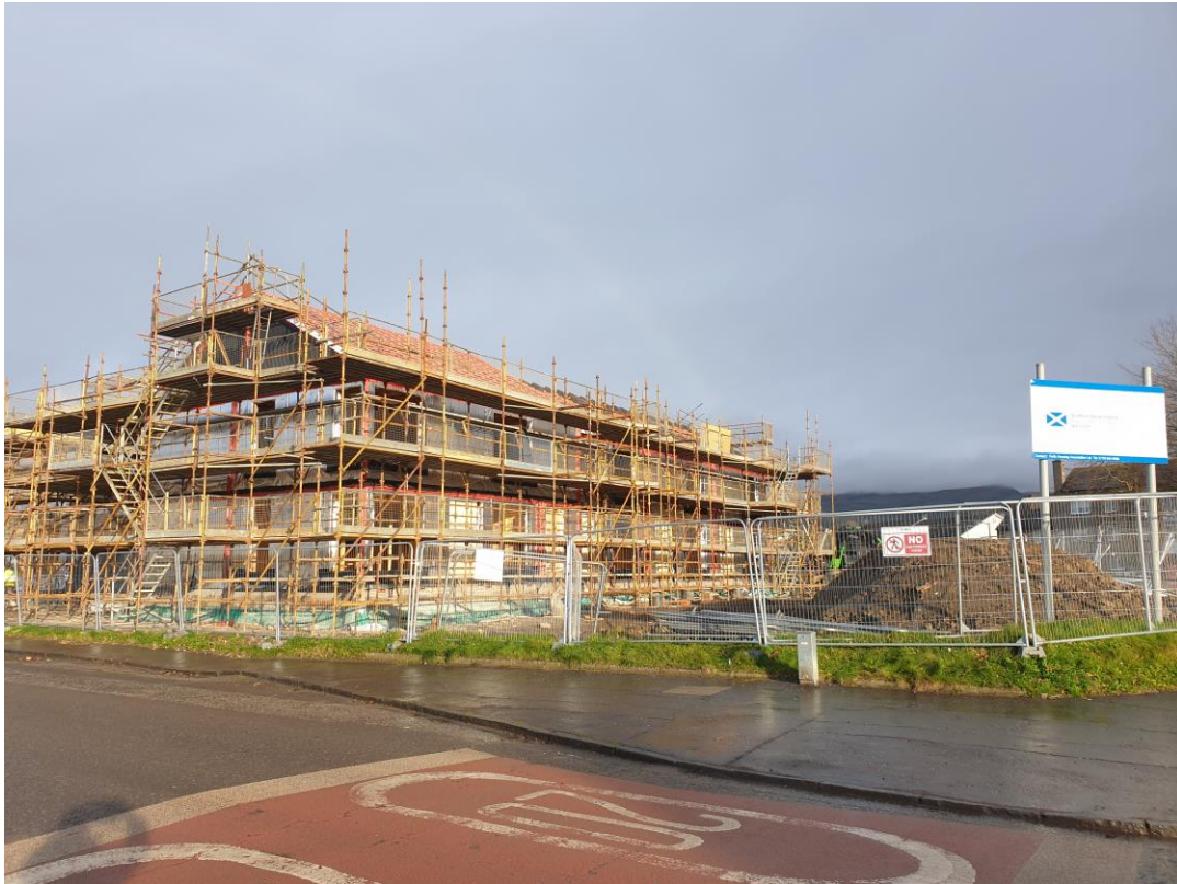
Housing under construction at Johnston Avenue (Phase 2), Cornton
